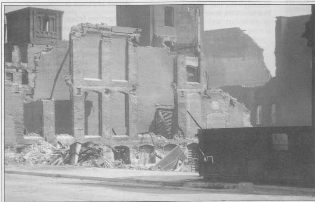
In August 1998, a wind-fed fire destroyed a city block of what was part of R.J. Reynolds' manufacturing complex in downtown Winston-Salem. Built in the early 1900s, the property was being renovated as part of the Piedmont Triad Research Park. Left: The interior wall of 256-1 on Chestnut Street. Below: #256-2 on Patterson Ave. The dark 'spot' below left center of the truck was a car. Photos courtesy Elizabeth W. Sapp.
