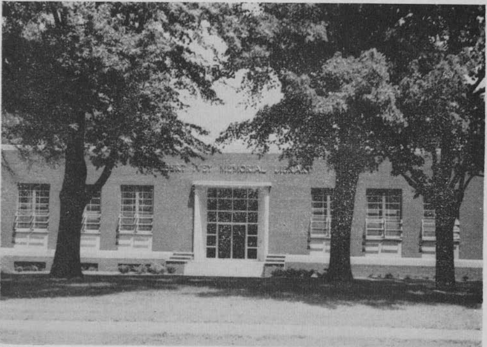
Elbert Ivey Memorial Library in Hickory. The new Library building, with a book capacity of 100,000 volumes was given to the city of Hickory by the family of the late George F. Ivey, as a memorial to Elbert A. Ivey (1900-1942). Of conservative modern design, the $130,000 building was opened to the public on March 29, 1952. The first birthday was celebrated.
