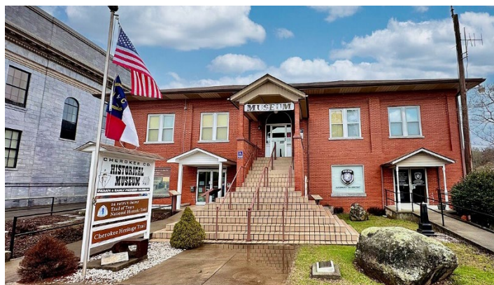
Murphy NC Carnegie Library. Source: The Murphy NC Carnegie library building now houses the Cherokee County Historical Museum - List of Carnegie libraries in North Carolina - Wikipedia.
