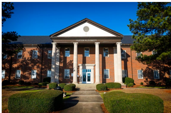
Clifton W. Everett building where PCC library is located
